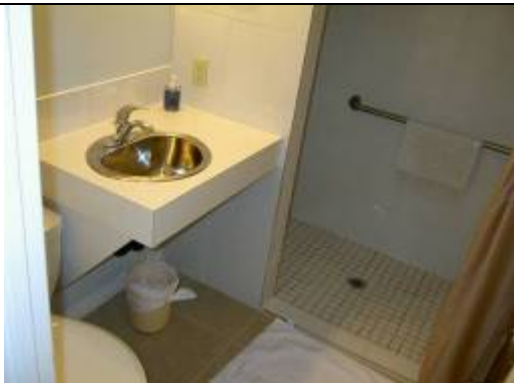
Wheelchair accessible shower/new sinks
